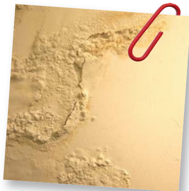
Figure 2: damage caused by untreated condensation
