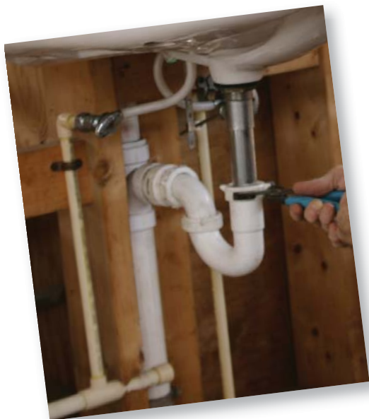
Figure 1: sink waste trap or u-bend
